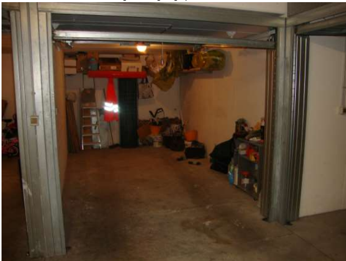
Fig. 8.26 – garage piano interrato
